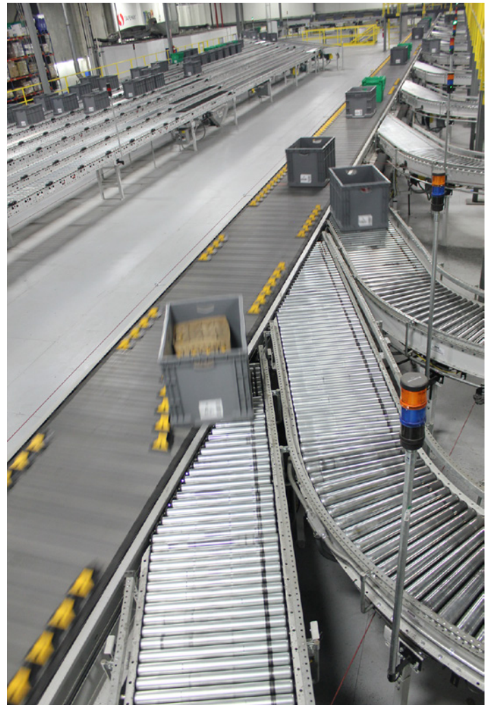
Inventory totes (gray) and retail store totes (green) are directed to Multishuttle sub-system on a sliding shoe sorter.
